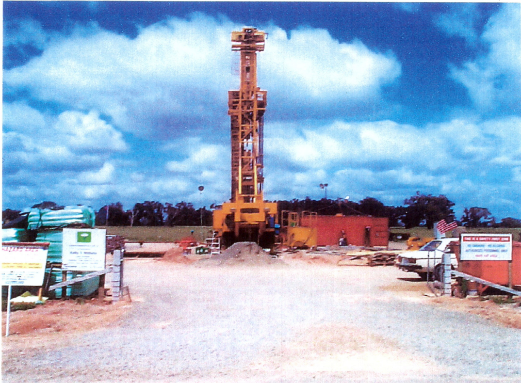
KELLY-1 VIEW OF RIG FROM ST JAMES ROAD
