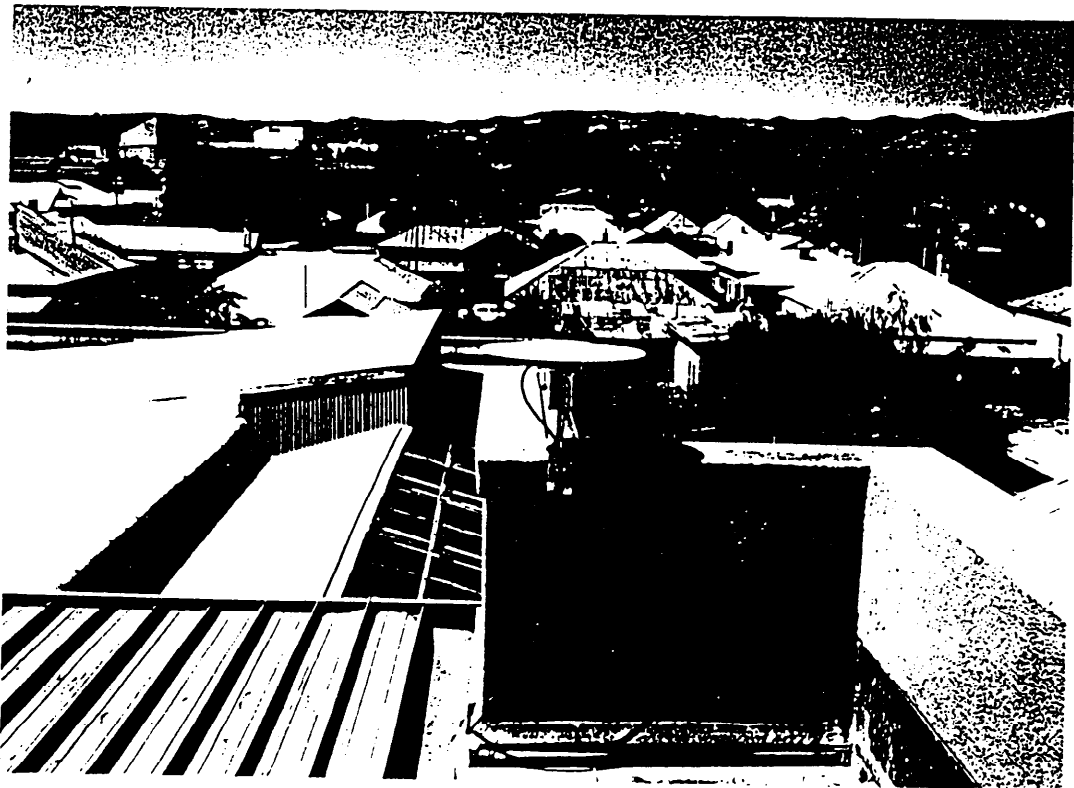
ADELAIDE ANTENNA LOCATION
